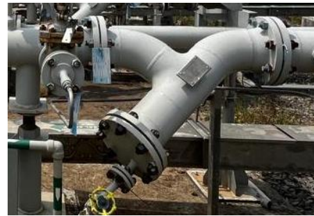
Gambar 4 Suction Strainer
