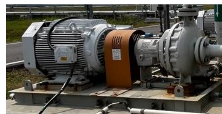
Gambar 6 Water Injection Transfer Pump Skid
