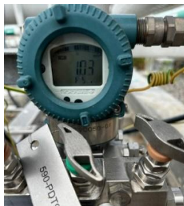
Gambar 3 Indikator Tekanan Diferensial Suction Strainer
